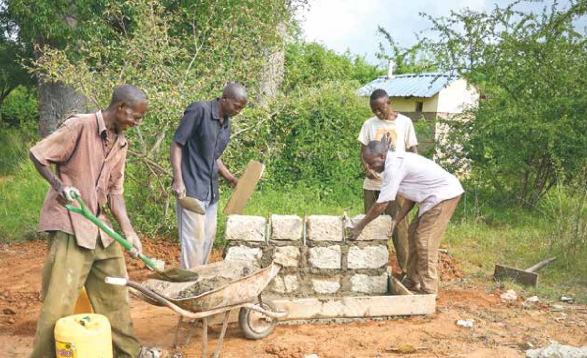
Workers put finishing touches on a water point at St. Michael the Archangel Church in Kamboo. The wider Kibwezi region has been devastated by climate change.
